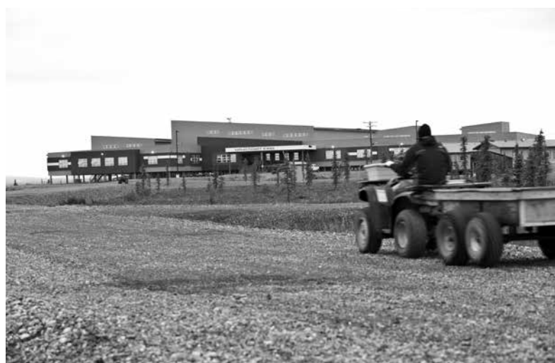
The Napaaqtugmiut School (K-12) in Noatak, Alaska, built in 2009. The building, like most in the region, is elevated above the ground to prevent its heat from melting the permafrost.
